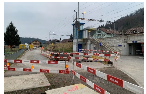
Rerouting of the mixed water pipe in the factory path
